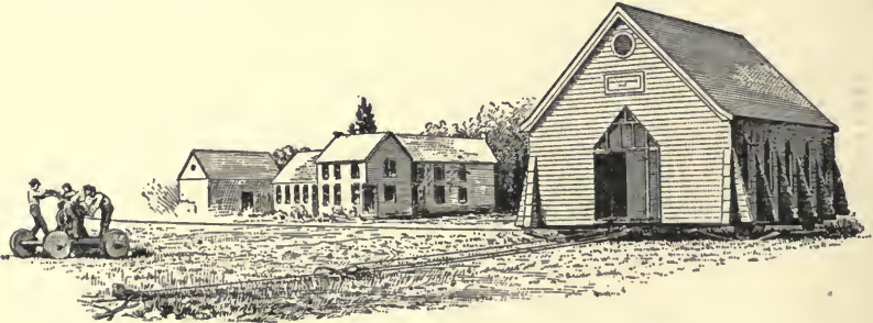
Fig. 141. Method of Moving Light Frame Buildings.
